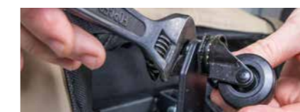
4.3.2 Attach castor stem through plare, lock in place with retaining nut
